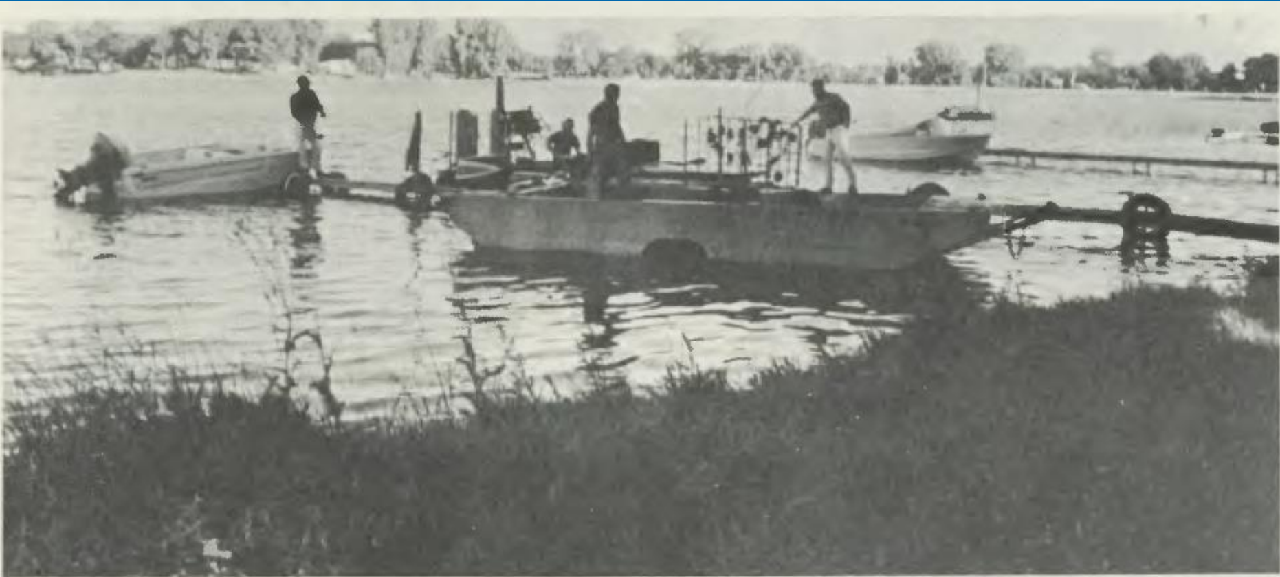
Chemicals applied from an airplane-propeller-driven barge replace the bed spring on Lake Awasso, St. Paul, Minn.
