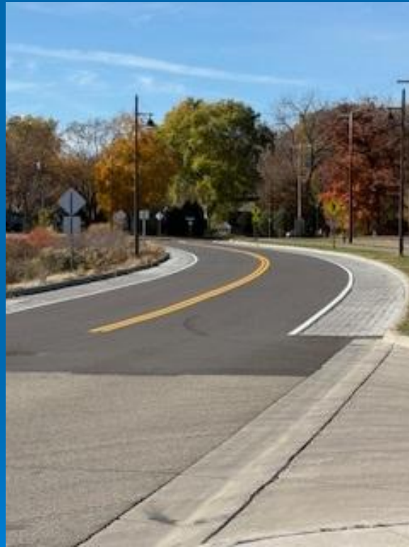
Looking west on North Owasso Blvd.
